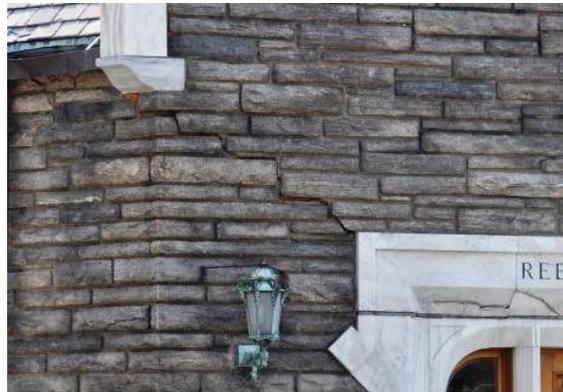
If you have been following our building restoration story you may recall that the lintel, the steel beam over the front doors on which the marble and granite rest, exhibits heavy rust and rust jacking. This is the primary cause of the cracks in the granite and marble over the entry doors.
